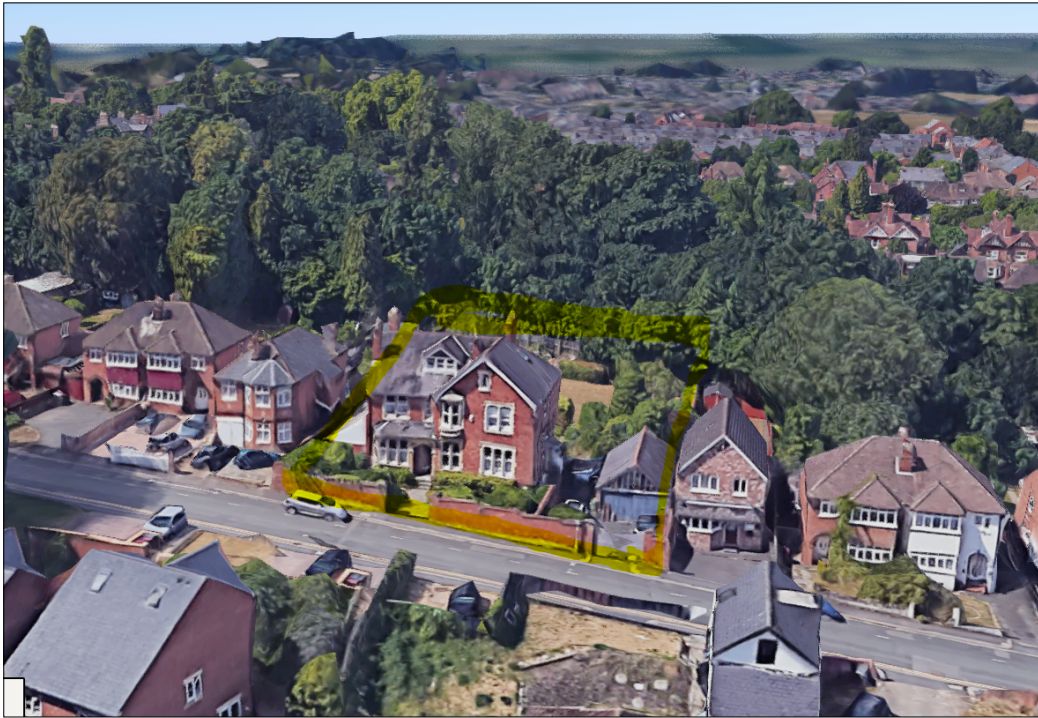
Fig 7: Aerial view (Google maps 2019)
